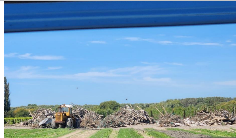
Mixed piles, that cannot be further separated.
