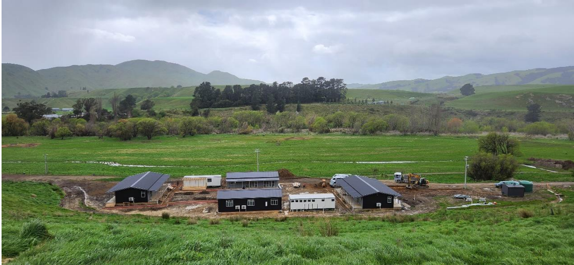
Figures 1 and 2: New seasonal workers accommodation at vineyard
