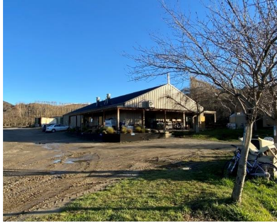
Figure 4.25: RSE accommodation facilities block at Dunstan Hills
